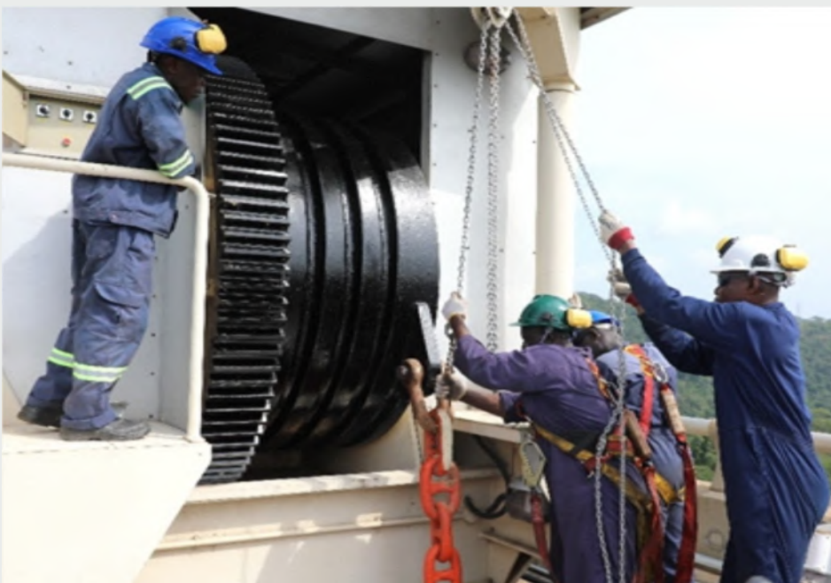
Some Staff working on the Spillway hoist control.
