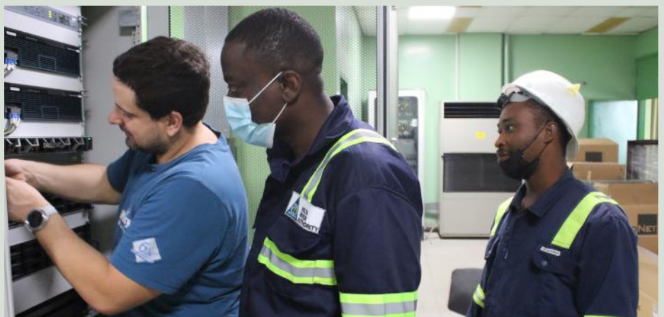
Replacement of SCADA servers
