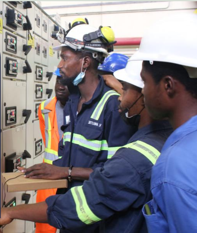
Replacement of touch panels
