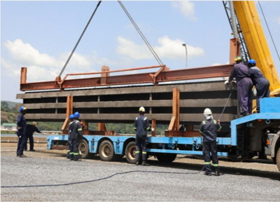
Transportation of spillway stop logs.
